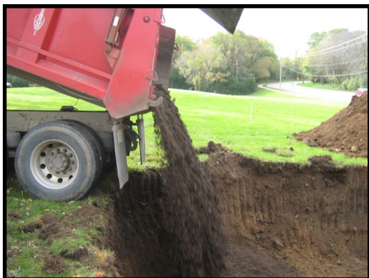
Installation of engineered soil mixture into excavated bioretention cell.
