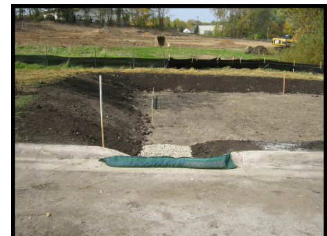
Bioretention cell with sediment control and blocked inlet to keep the cell off line during establishment
