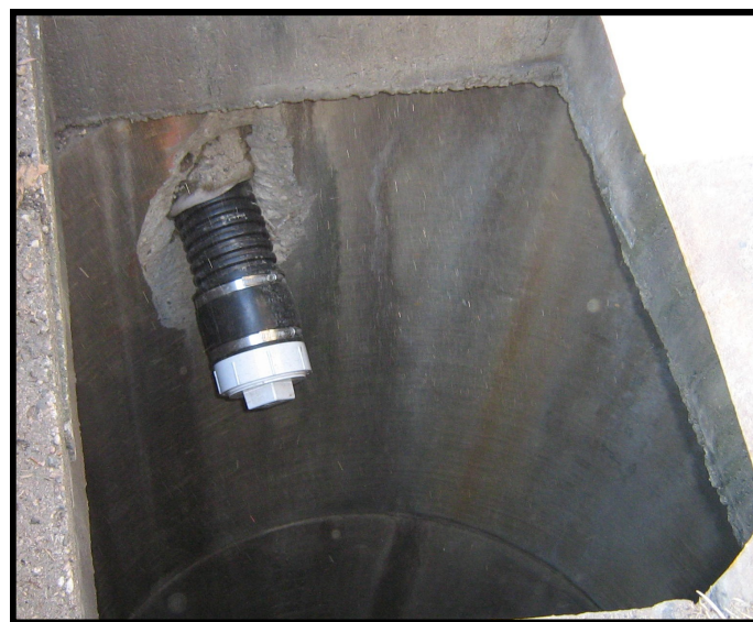
Accessible under-drain outlet for a bioretention system to adjust residence time within the bioretention cell
