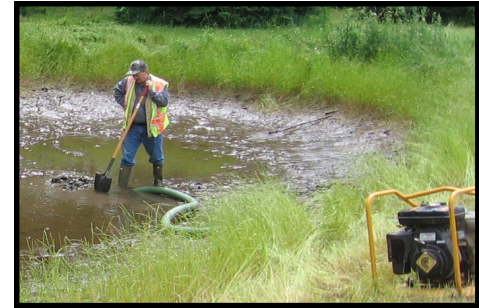
Excess water and sediment should be removed prior to excavation
