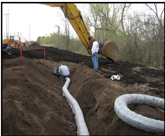
Installation of an under-drain system in a bioretention system
