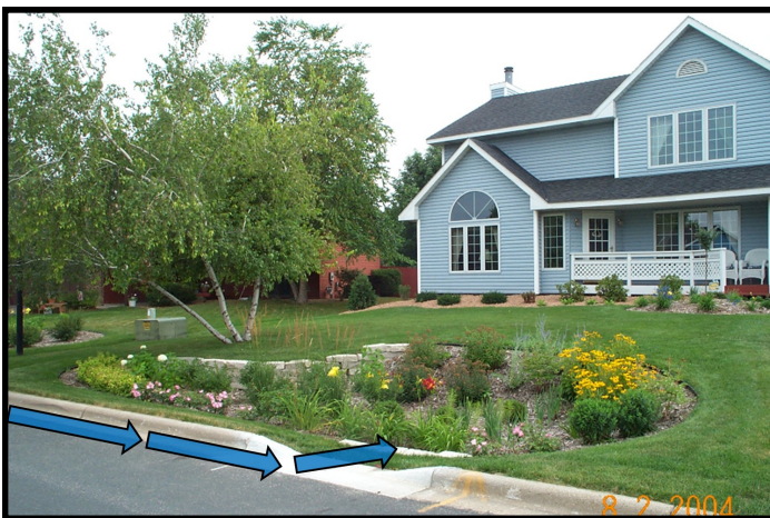
Off-line cell design during low flow
