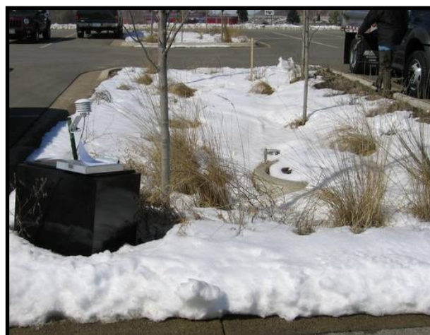
Cottage Grove Bioretention Cell Cottage Grove, MN
