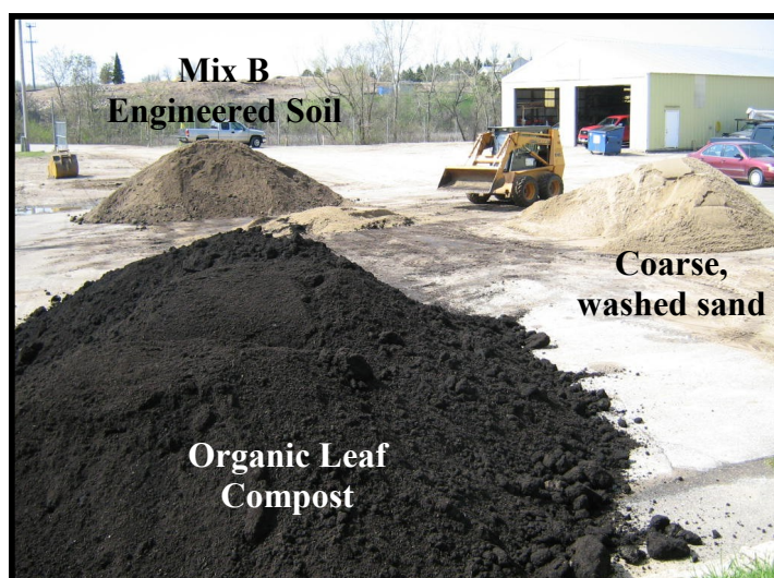
On site mixing of engineered soils
