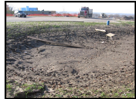
Non-functional bioretention cell due to construction sediment damage
