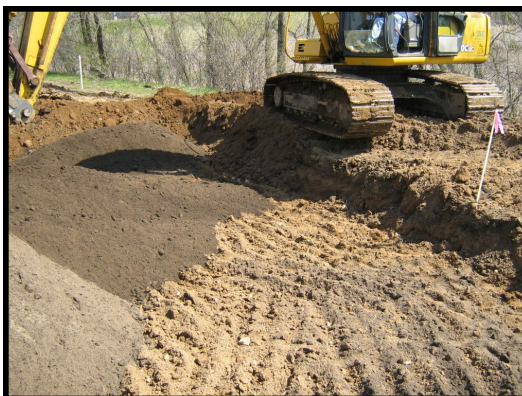
Engineered soils placement on flat and level excavated cell bottom
